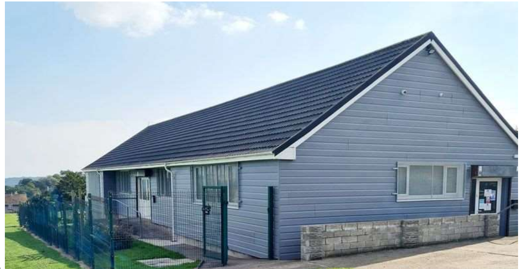
Bryntirion & Laleston Community Centre after Cladding
