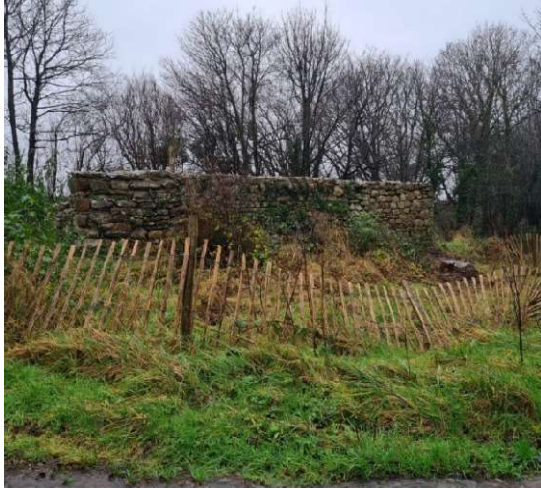
The Pound before renovation
